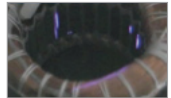
Corona discharge in motor
